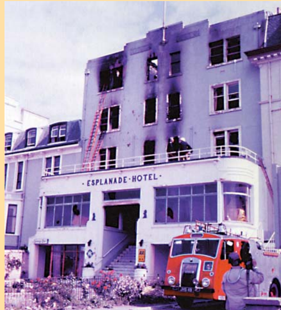
The fire gutted The Esplanade Hotel, Oban, in 1973 in which 10 people died.
